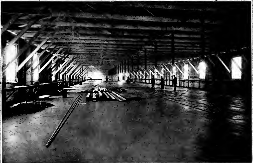
The plate shop at the Hanlon yard is a light, roomy structure; each tool being surrounded by a wide expanse of floor space. The mould loft is arranged with high ceiling giving a large amount of storage space overhead.
